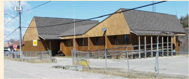
Pic River Elementary School Heron Bay
